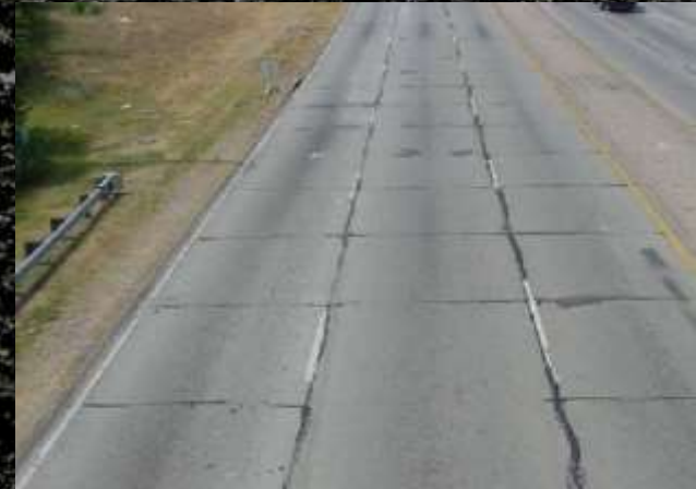
Reflection cracking
