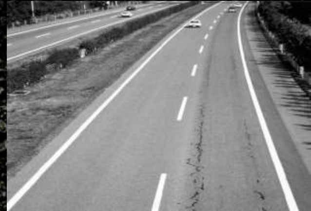
Top-down cracking
