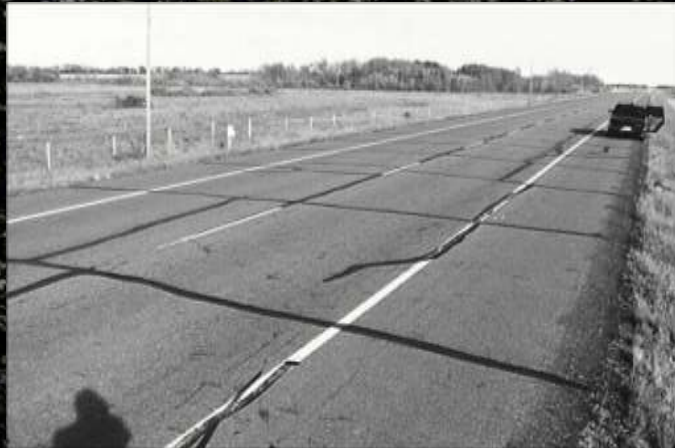
Transverse cracking
