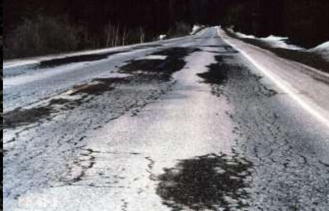
Bottom-up cracking
